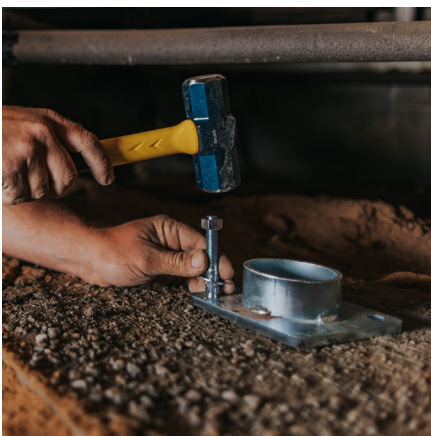
Anchor bolts installed into concrete footer.
