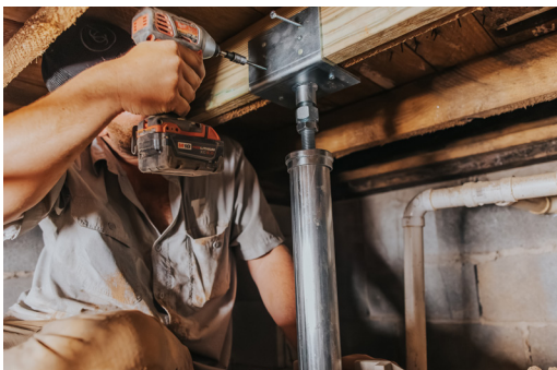
Attaching saddle bracket to block and single joist.
