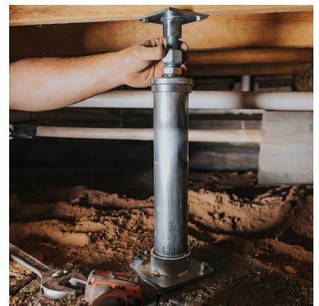
Assembled system on concrete footer.
