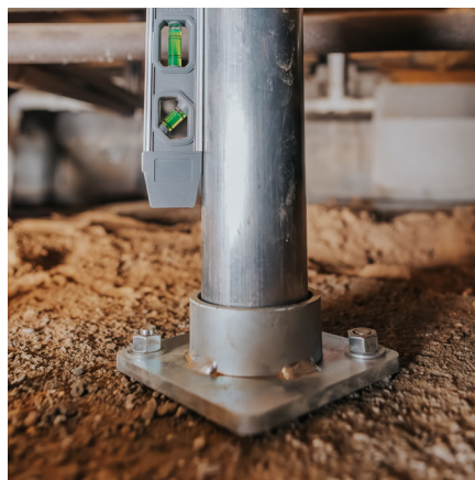
Base Mount installed on concrete footer.
