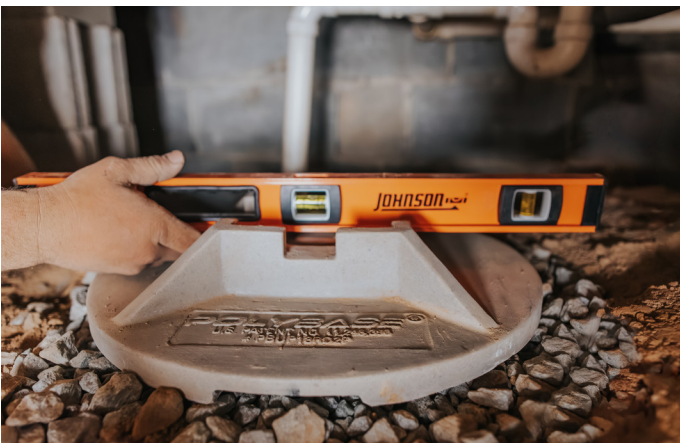
PolyBase® installed on 57 stone.
