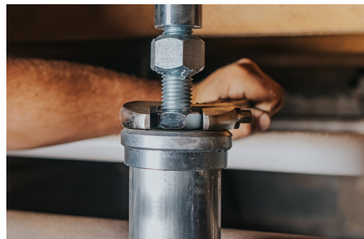
Tightening adjusting jam nut.
